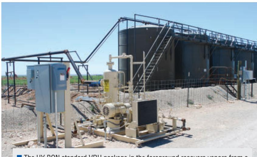
■ The HY-BON standard VRU package in the foreground recovers vapors from a multiple oil storage tank battery at an Eagle Ford Shale site in south Texas.
