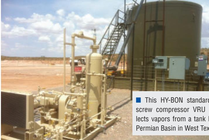
■ This HY-BON standard oil flooded screw compressor VRU package collects vapors from a tank battery in the Permian Basin in West Texas.
